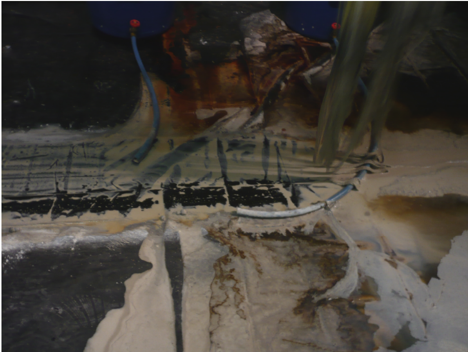
Fig.3.10: Leaking fluids. ON TRACK at Thessaloniki Biennale. May 2009. © in serial .
