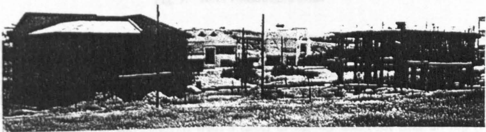
Fig. 7. Private dwellings in the construction stage.
