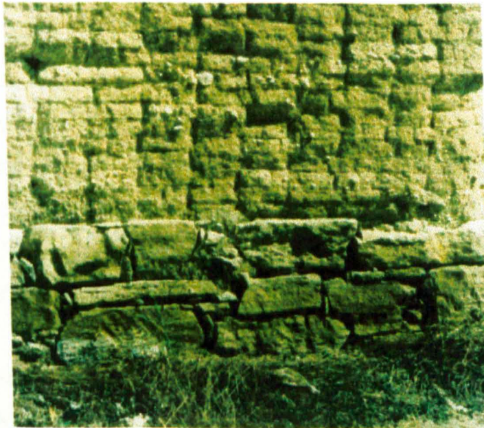
Figure 2.4. Stone blocks were used for the wall foundation.
