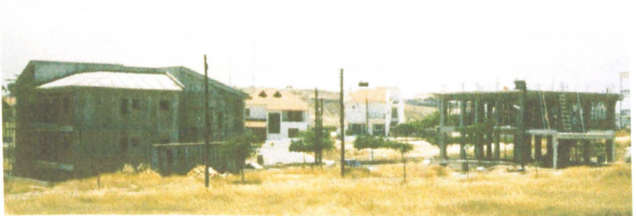
Figure 2.9. Private dwellings at the construction stage.
