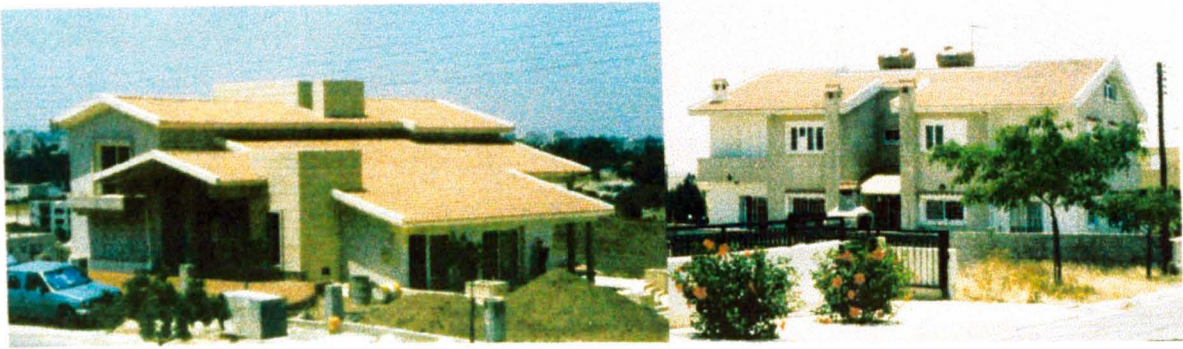
Figure 2.12. Inclined concrete slabs covered with roof tiles.
