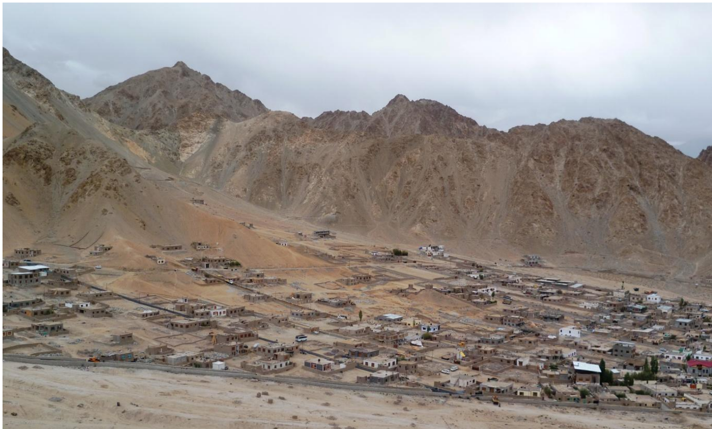
Figure 4.4 Recent constructions on barren land in the margins of Leh town (Le Masson, 2011)
