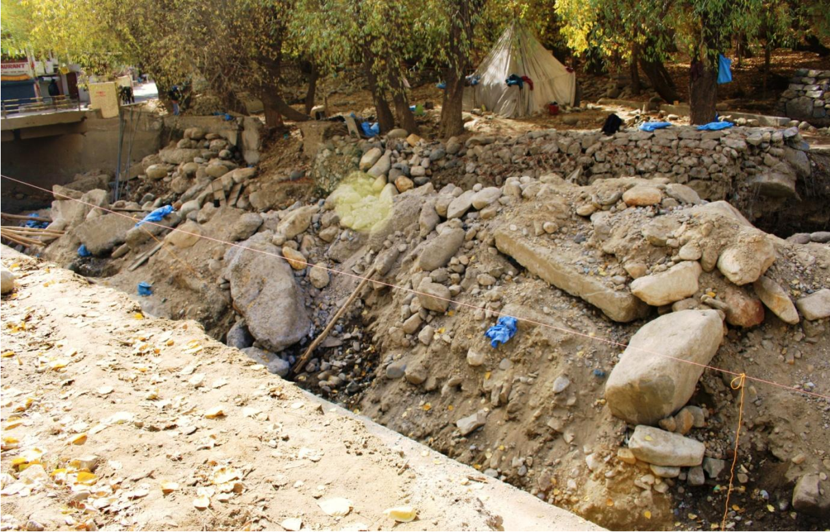
Figure 7.4. Remains of the road downstream along the same river one month after the floods (Le Masson, 2010)
