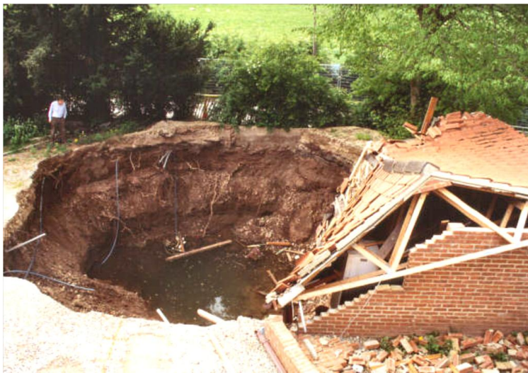
Fig. 2.8: Sinkhole at Ure Bank Terrace, Ripon-UK (from Cooper, 2006); the hole formed in April 1997, 10m across and 5.5 m deep. It was caused by collapse of a cave formed in Permian Age gypsum.
