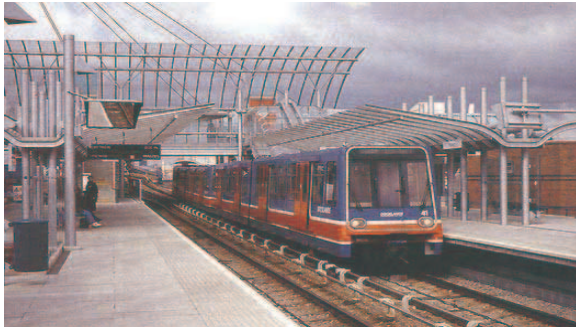
Figure 2.5.1 – Docklands Light Railway
