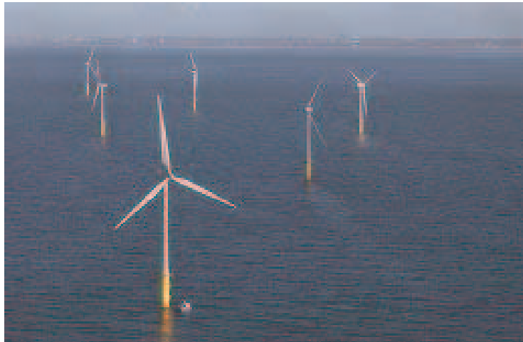
Figure 29 - North Hoyle offshore wind installation
