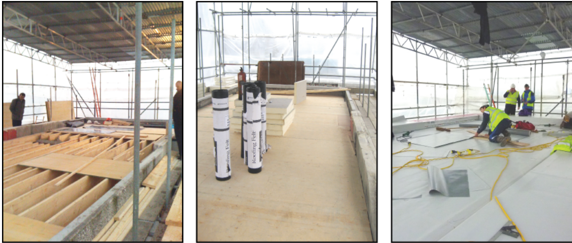
Figure 5.27 Steps taken during roof renewal.
