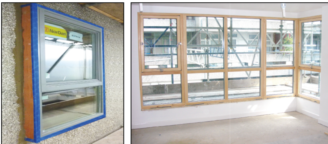
Figure 5.28 New triple glazing (with an internal view from the living room).
