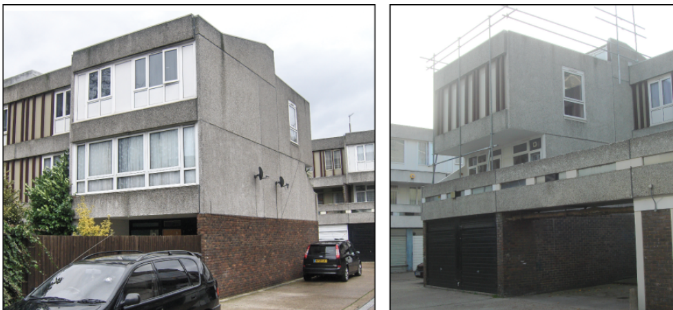
Figure 5.1 Photographs of the South-West and North-East elevations prior to retrofit works.
