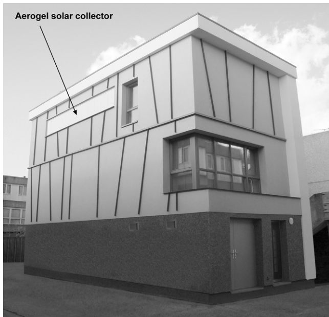
Fig. 8. South-east elevation of the retrofit house.
