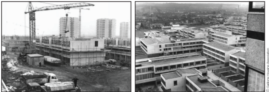
Figure 5.2 Historic photographs of the Thamesmead estate being constructed.
