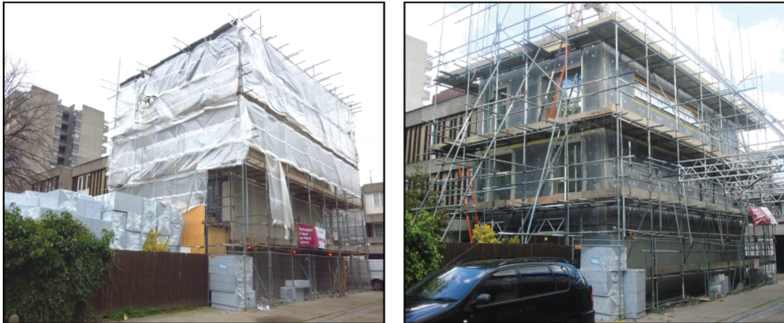
Figure 5.33 External insulation during and after installation.
