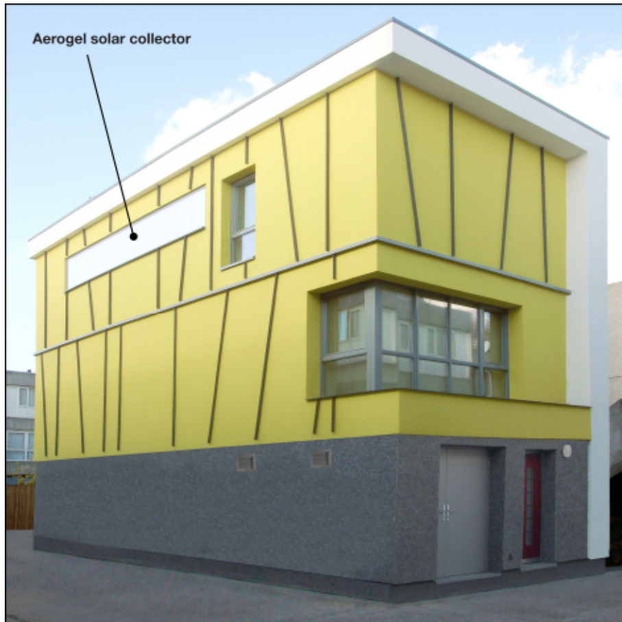
Figure 6.10 South-east elevation of the retrofit house.
