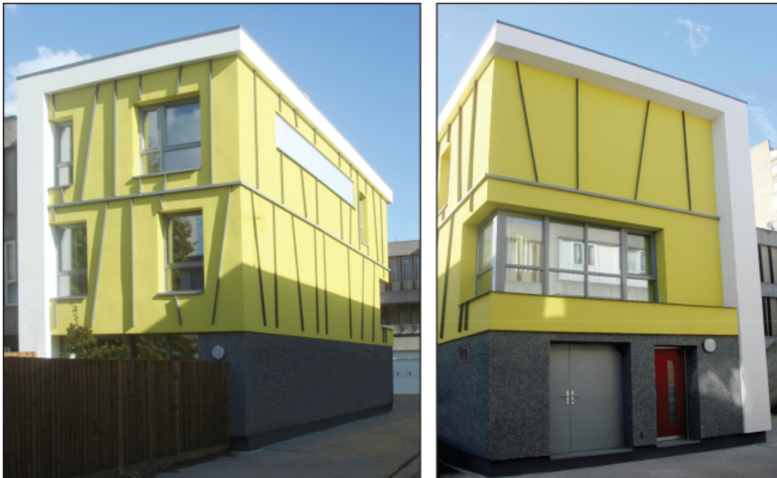
Figure 5.39 Photographs of the completed retrofit house.
