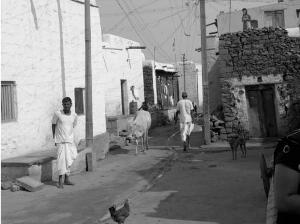
Figure 2: Energy infrastructure running along the row houses in Ilkal region
