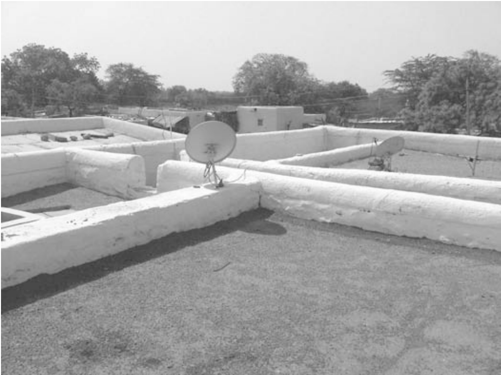
Figure 3: Flat roofs spanning 15 houses in Ilkal region
