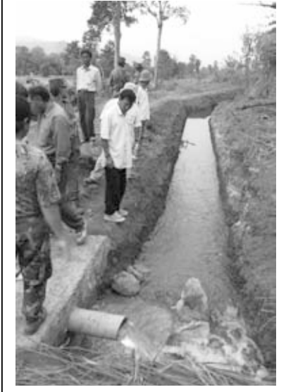
Figure 4: Part of the 30 km irrigation canal that was constructed in 10 days
