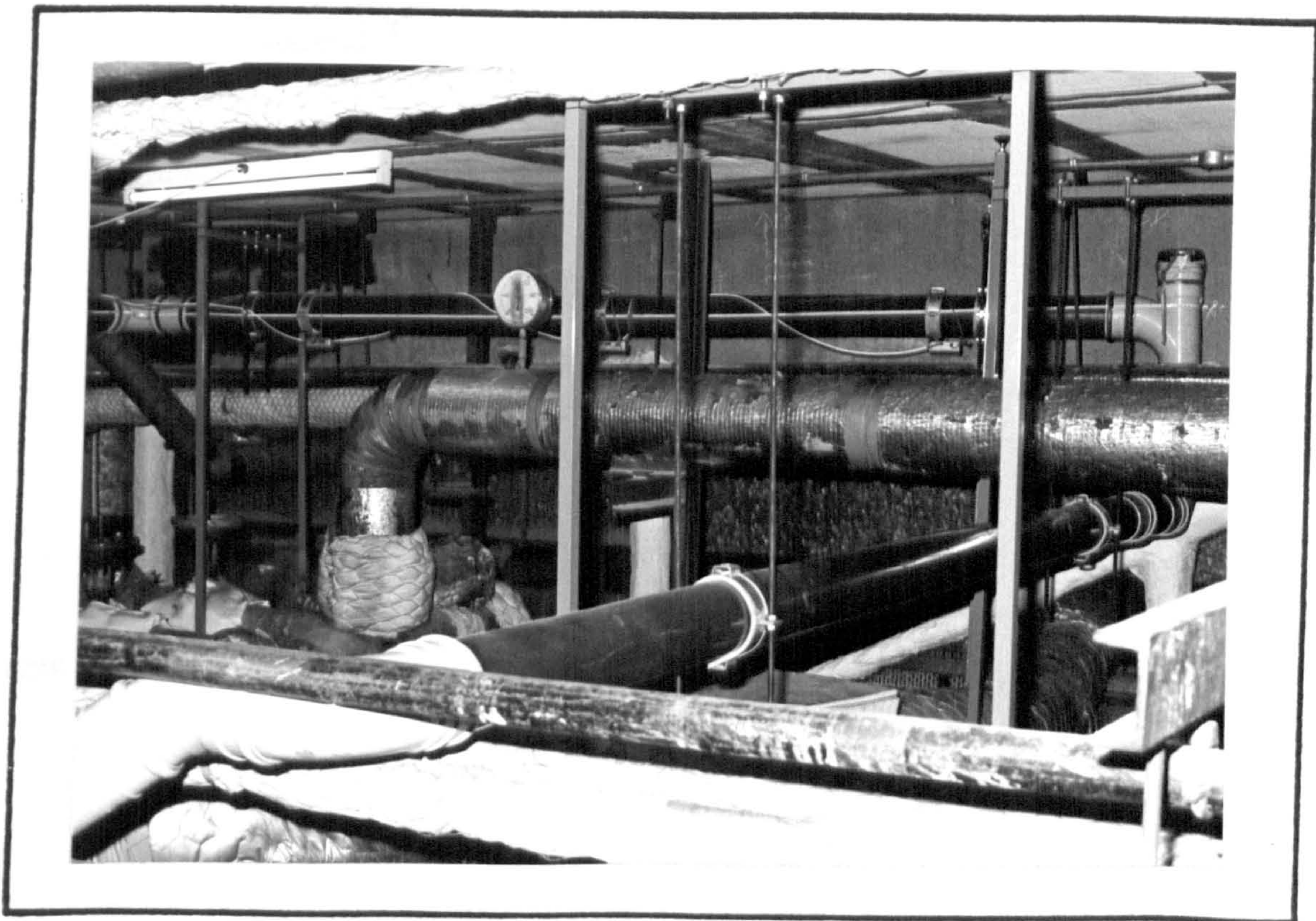
FIGURE 9/13. - General View of Installed U.P.V.C. Service to the Male Facility.
