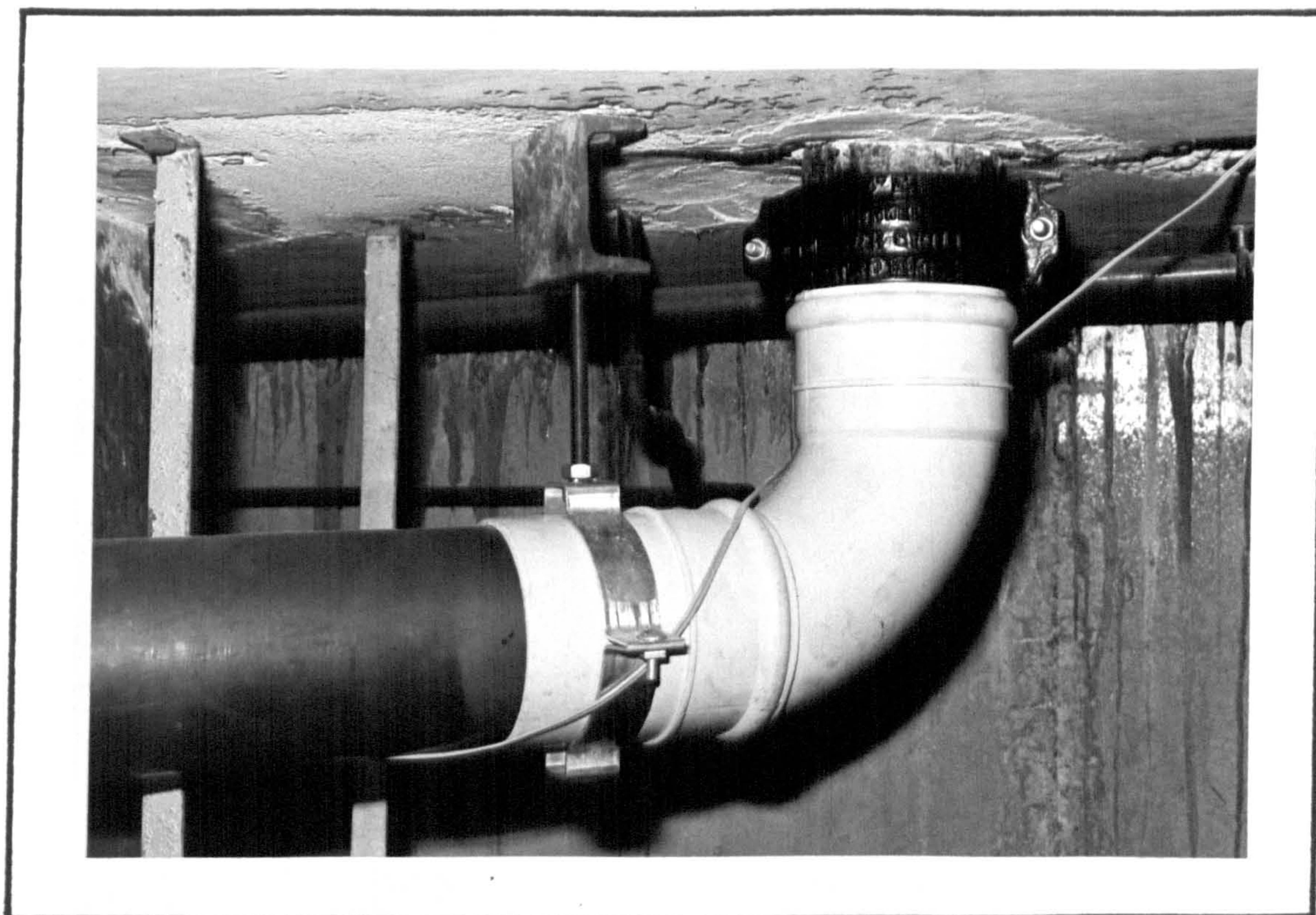
FIGURE 8/1. - Inlet to Discharge Pipe, ('On-Site').
