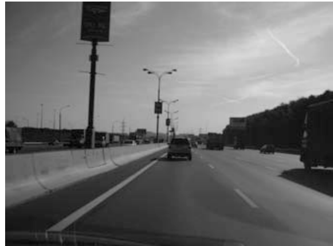
Figure 5. Typical City Road (Moscow)
