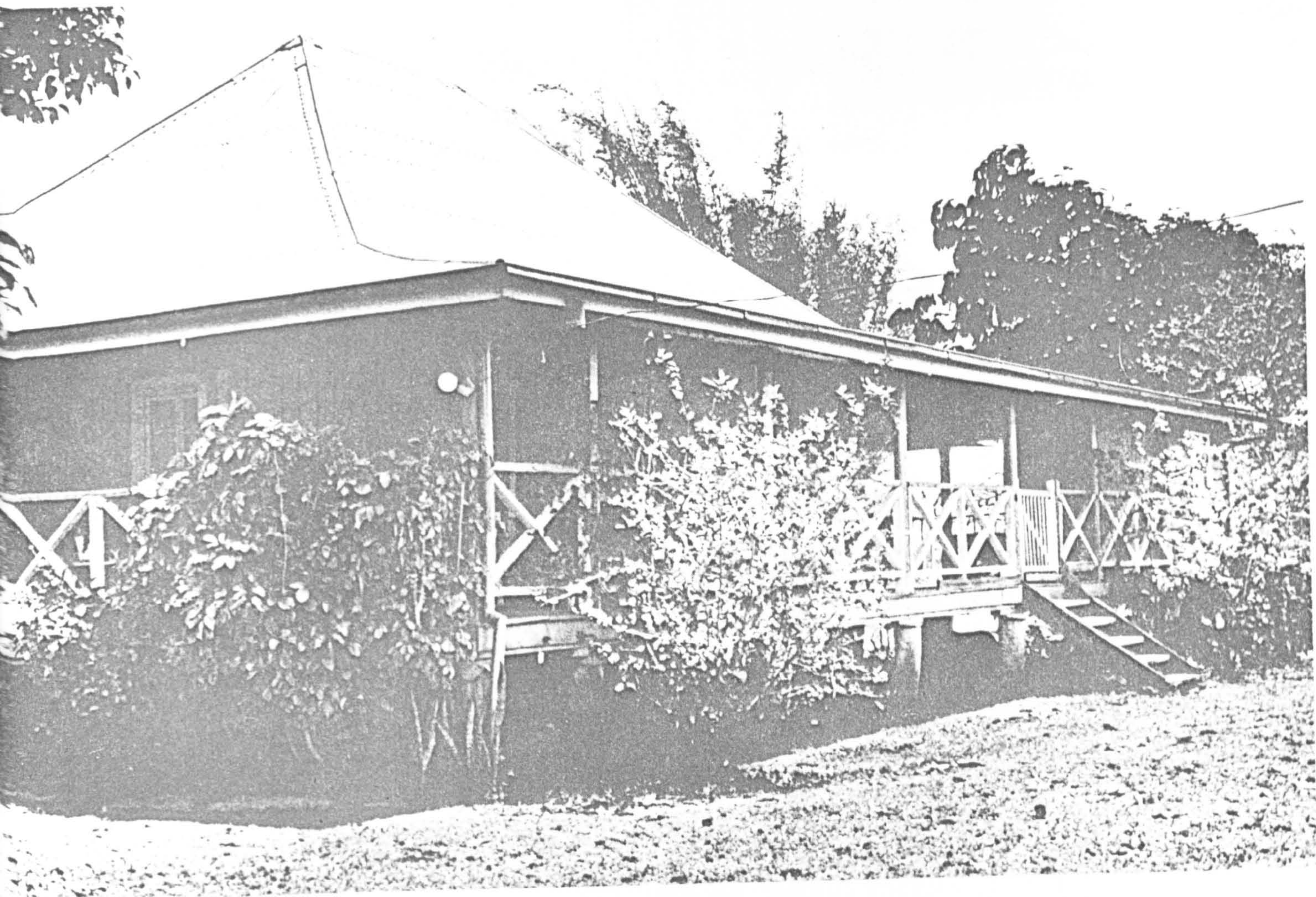
Inkerman, built in 1870 of pitsawn timber. Old telegraph repeater station at far end of verandah.
