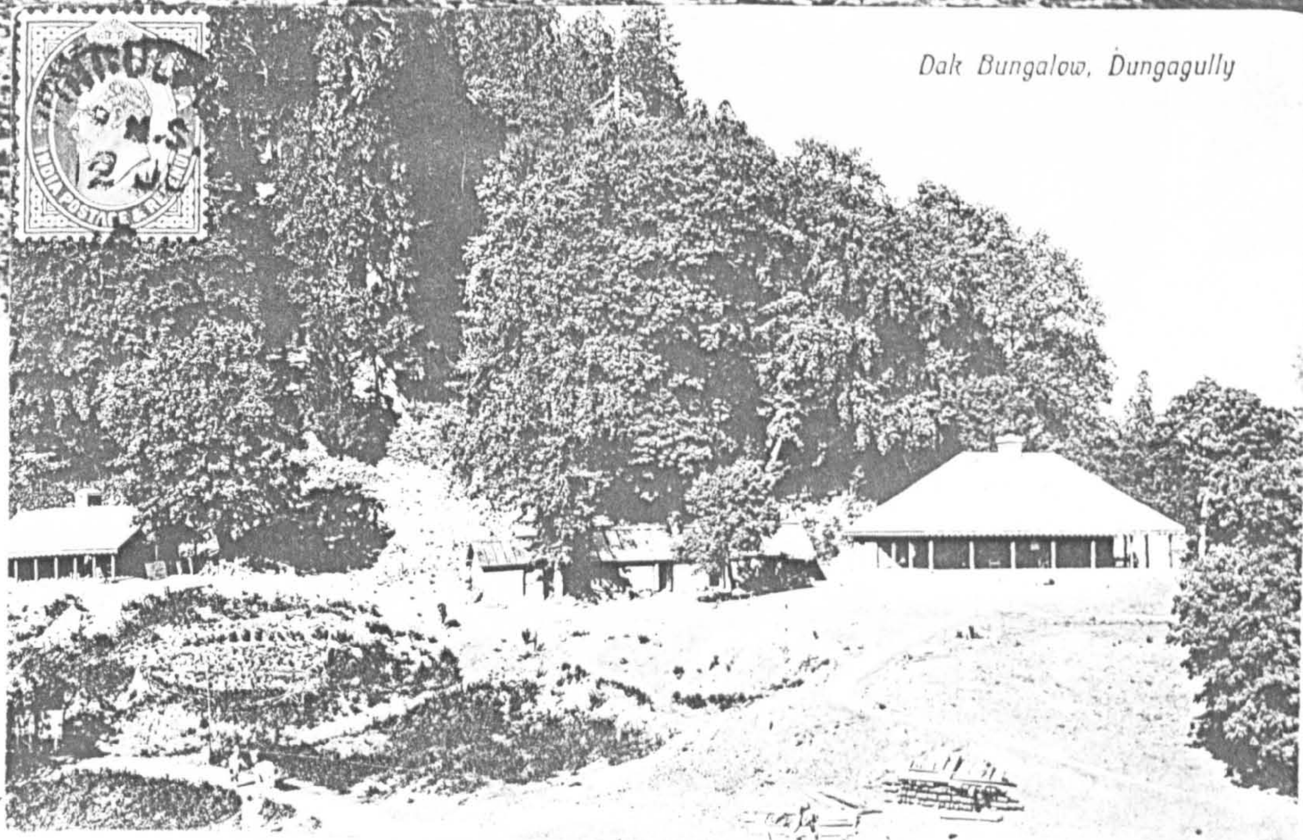
The dak bungalow c1850 F.Fiebig (Courtesy IOL) 1968 (ADK) c1912
