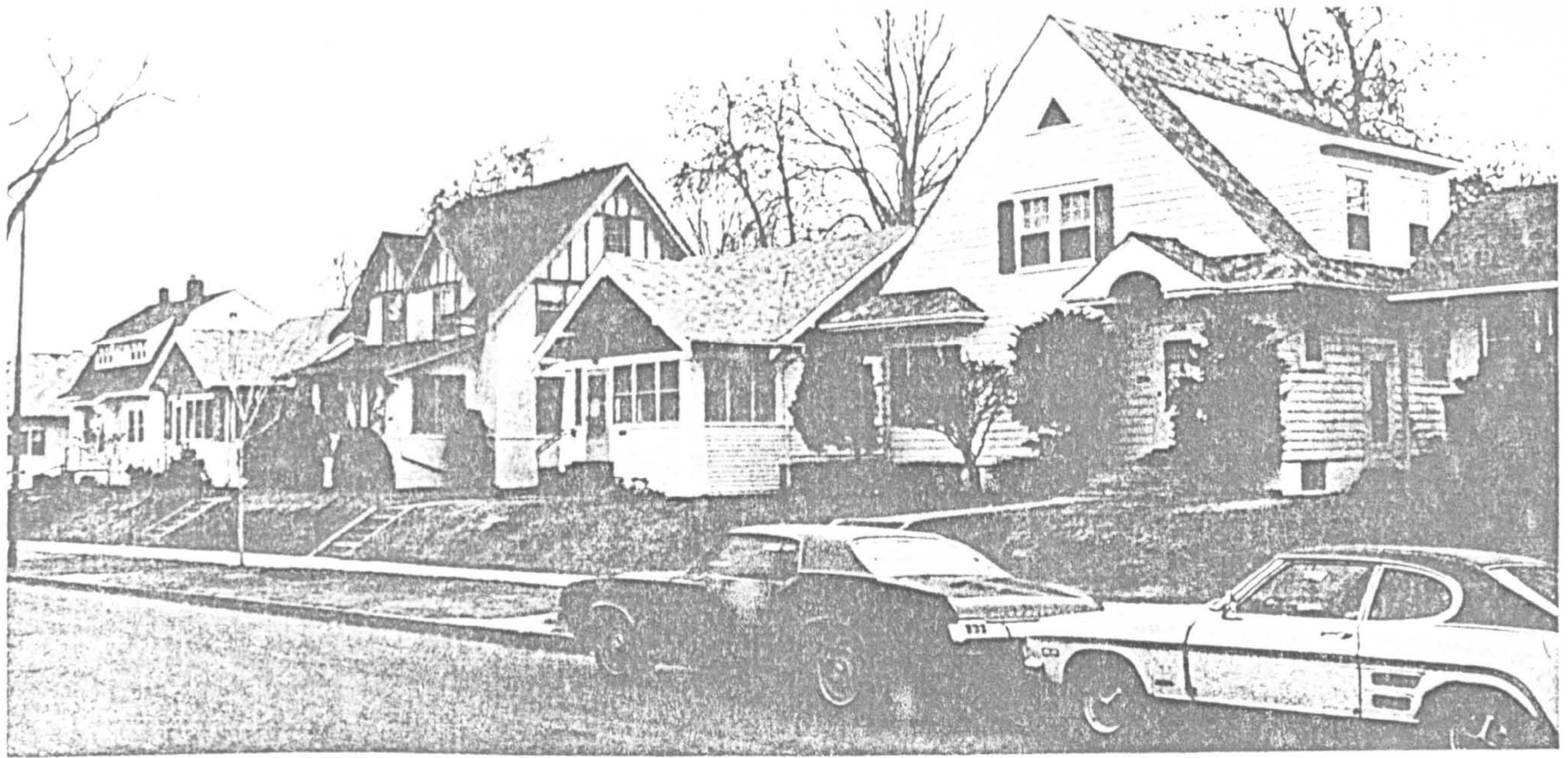
During the 1920s real estate developers sometimes built groups of bureau-designed homes. In this block three A.S.H.S.B. houses stand on alternate lots—a two-story Dutch Colonial, a half-timbered English, and a Colonial. The two bungalows between are not bureau designs. St. Paul, Minnesota, 1980. Photograph by the author. The weekly newspaper column written by the A.S.H.S.B. popularized some unusual styles, such as the airplane bungalow, which brought diversity to suburban developments throughout the country.
