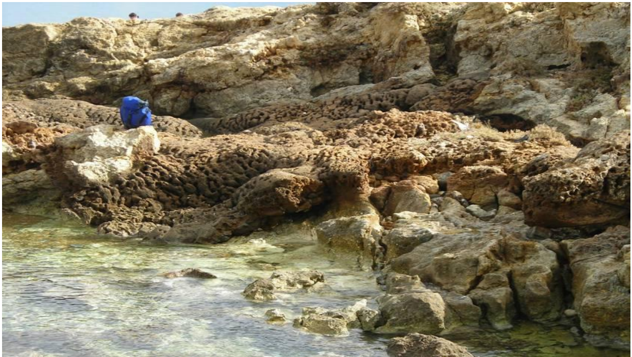
Figure 4.1.8: The uplifted dead trottoir undercut by small notch at present sea level.
