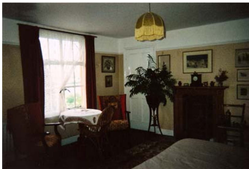
Figure 6.8 The 1950s window. Next to the window on the right is the great bolt painted in white. The bolt was installed in the 1950s for safety reason and was used by people to hoist themselves out of the window in the event of fire.
