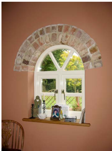
Figure 6.33 One of the features, the brick window arches, that the coach house is required to maintained.
