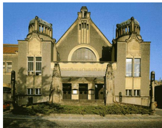
6 The National House Prostějov main façade 1905-07
