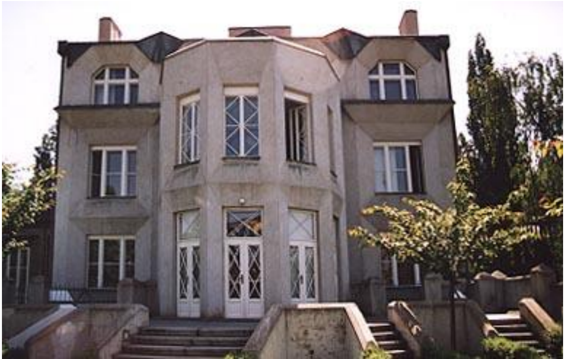
1 Front elevation, recent photograph with mature gardens
