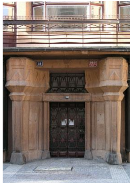
3 The imposing doorway with Cubist columns and metal, glass panelled door
