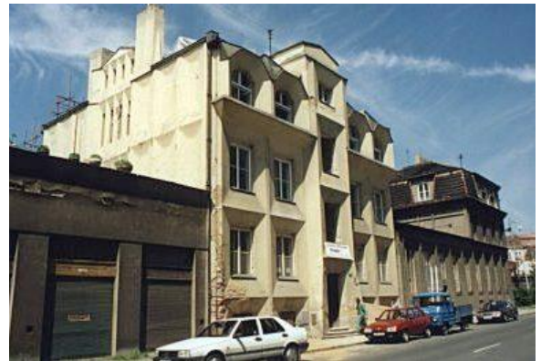
3 The significantly reduced height of the rear elevation testifies to the drop front to back
