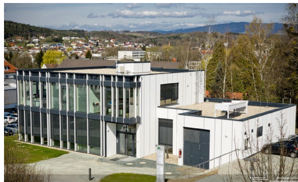
Figure 3. External photo of the case-study PRELUDE pilot building
