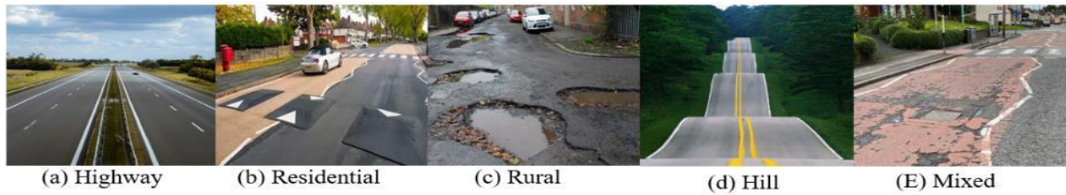
Figure 4.7 Road profiles categorised according to the prevailing road conditions.
