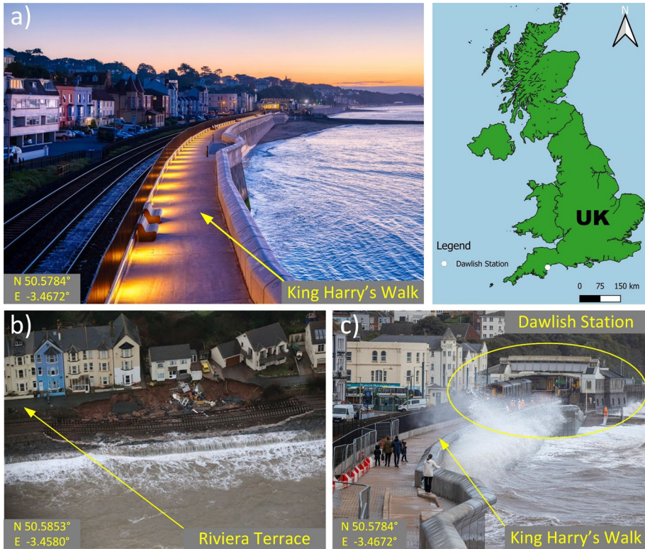
Fig. 1 Location of Dawlish railway station. a The completed section of the new seawall looking towards the train station along King Harry’s Walk (Completed first section of Dawlish seawall at dusk (networkrailmediacentre.co.uk)). b An aerial view of the seawall damage sustained at Riviera Terrace in February 2014 (Dawlish aerial view of 2014 damage (networkrailmediacentre.co.uk)). c Waves impacting the newly constructed seawall south of the station, now 2.5 m taller with an integrated wave return (The completed first section of new seawall effectively deflecting waves back out to sea (networkrailmediacentre.co.uk))
