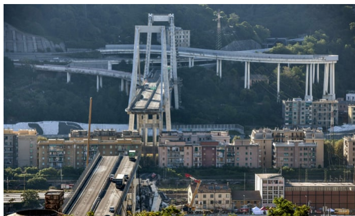
Figure 1.3: The Morandi Bridge (Genoa Bridge) Tragedy [15]
