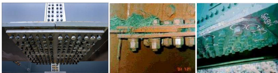
Figure 2.10: Preloaded and Loosened Bolting [29, 33]
