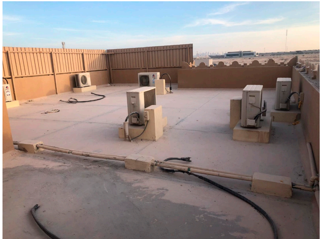
Figure 5. Example of a surveyed home roof.
