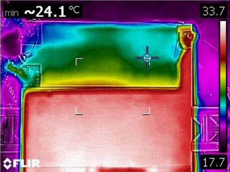
Figure 6-70. Detailed infrared imaging of the front heat pipe surface
