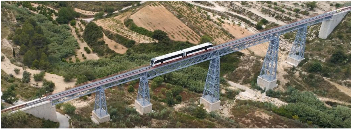
Fig. 1. Bridge view from a drone.
