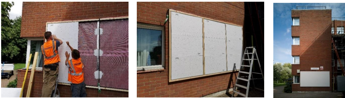
Figure 6: Stages of VIP installation at Brunel demo building.
