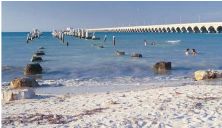
Fig. 2.5: The Progresso Pier in Mexico (Nickel Institute, 2018).
