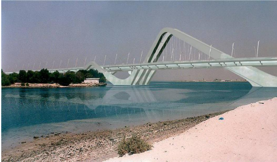
Fig. 2.7: Sheik Zayed Bridge in Abu Dhabi (Edvardsen, 2008).
