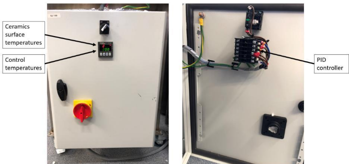
Figure 3-9 PID temperature control system electrical connections
