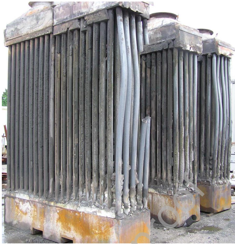
Figure 36: Corroded and fouled recuperators from an Aluminium melting furnace, taken from [99].
