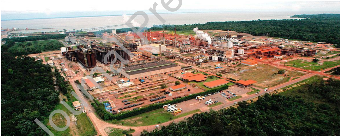
Figure 3: An aerial view of the largest alumina refinery, Alunorte. Reproduced from [43].
