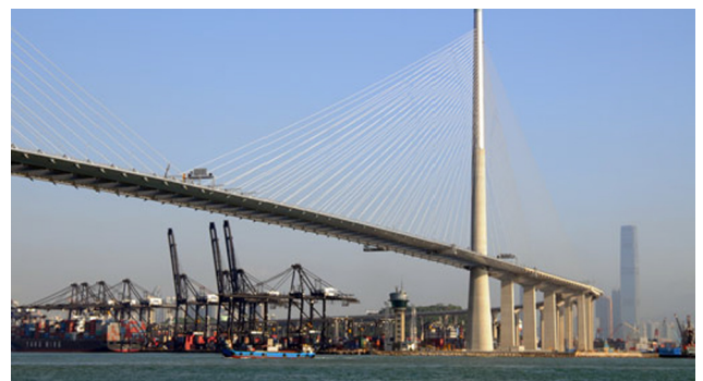
Fig. 2. Stonecutters bridge in Hong Kong [22].
