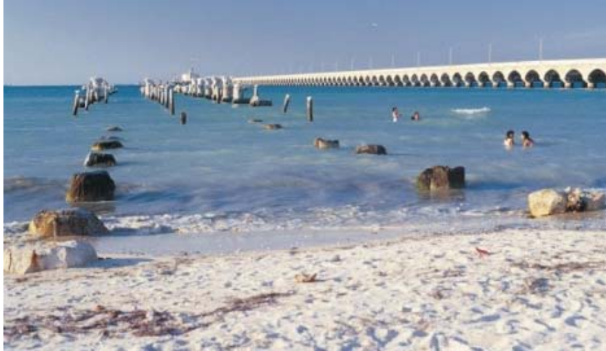
Figure 1 Progreso Pier, Mexico – the pier in the background was constructed in 1940 and used stainless steel reinforcing bar whereas the pier in the foreground was constructed in 1969 and used carbon steel reinforcing bar (Courtesy of the Nickel Institute)
