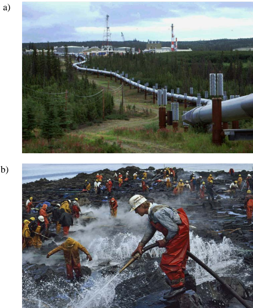
Figure 1-1a) Trans-Alaskan pipeline, USA [2], b) Clean-up efforts after failure [3],
