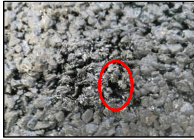
a) Missing aggregate on OPEN SMA surfaces
