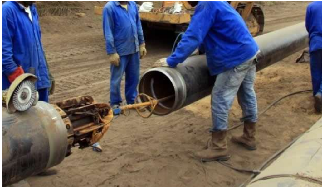
Figure 1.1. Example of a pipeline and laying maintenance by introducing a device inside the pipe.
