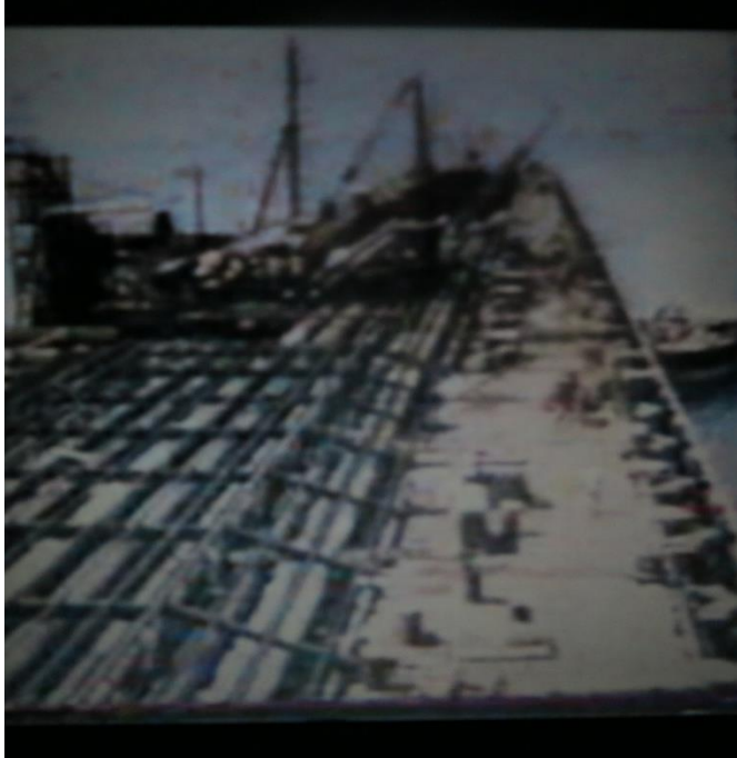
Figure 8. The construction of harbor (Wave,
