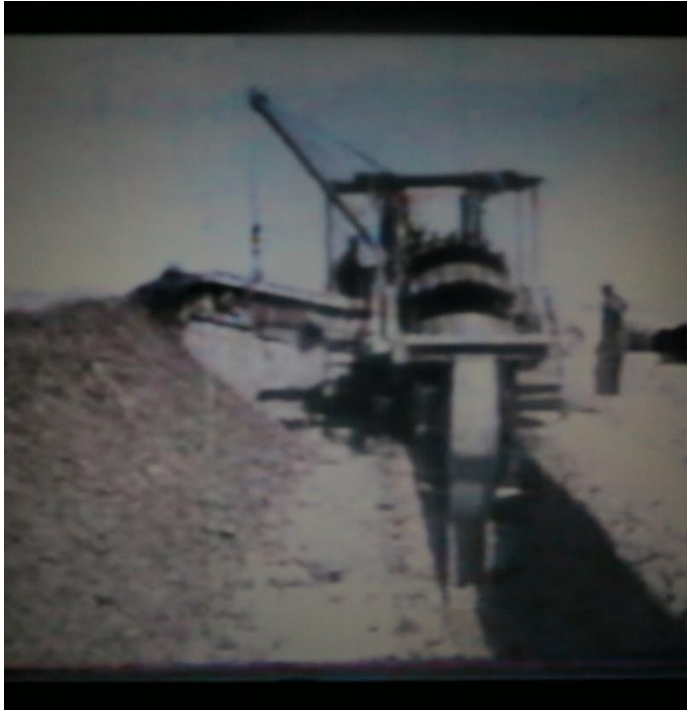
Figure 12. Preparing the pipeline's location
