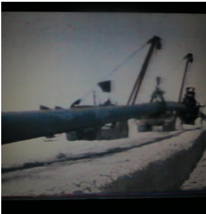
Figure 13. putting pipeline in their place
