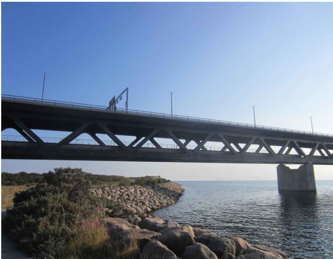
Figure 2-1 The Oresund Bridge at Malmö, Sweden
