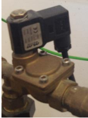
Figure 3. 19 Solenoid valve
