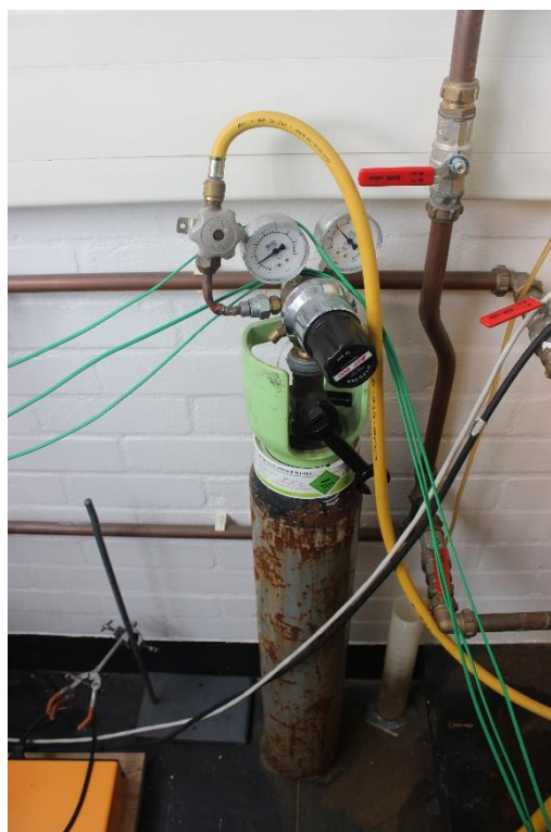
Figure 3. 7 Nitrogen gas cylinder
