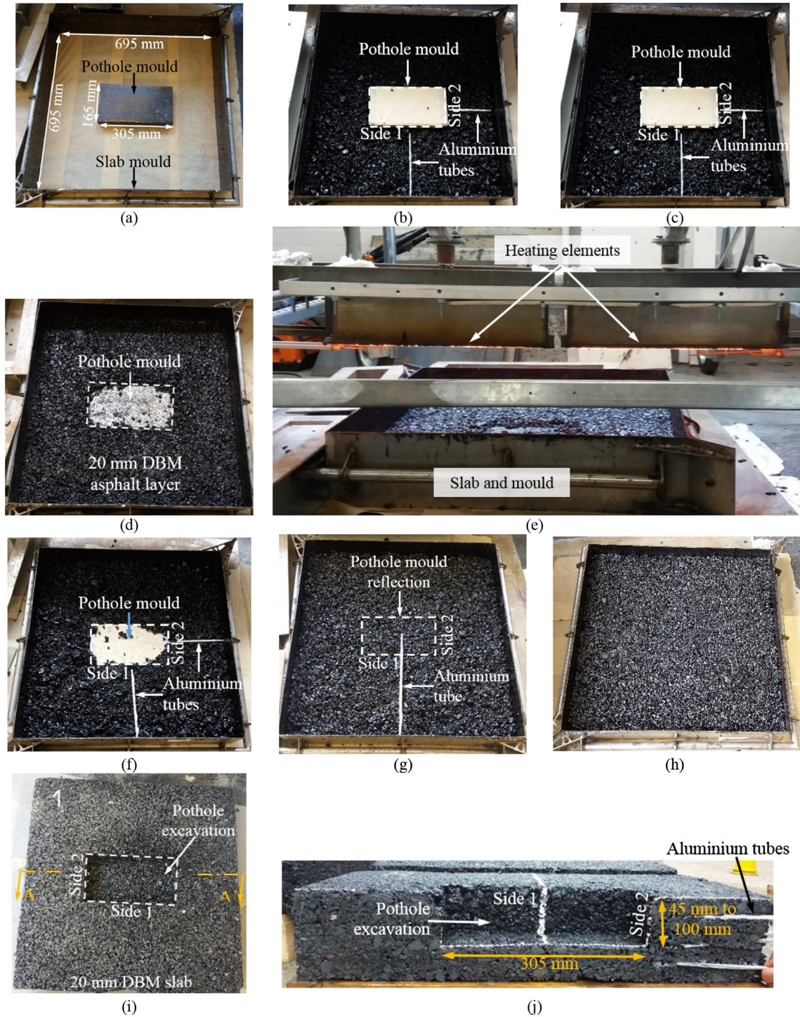
Fig. 2. Slab construction with embedded aluminium tubes to accommodate thermocouples for thermal tests: (a) moulds set up; (b) and (c) 4 aluminium tubes between six asphalt batches of first lift; (d) compacted first lift; (e) pre-heating of compacted lift; (f) and (g) 3 aluminium tubes between six batches of second lift; (h) compacted second lift; (i) slab turned upside down and pothole mould removed after 19 h of construction; (j) slab section A-A'.
