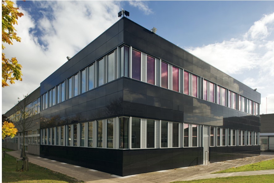
FIGURE 3.1: External view of the zero2020 testbed envelope upgrade
