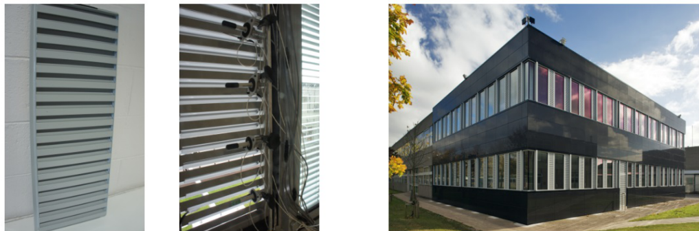
FIGURE 3.19: Left: Louvre module used for testing. Middle: louvre opening. Right: External facade of the testbed building showing the pre and post retrofit (see www.zero2020energy.com for more details). Integrated vertical slotted louvre banks also visible
