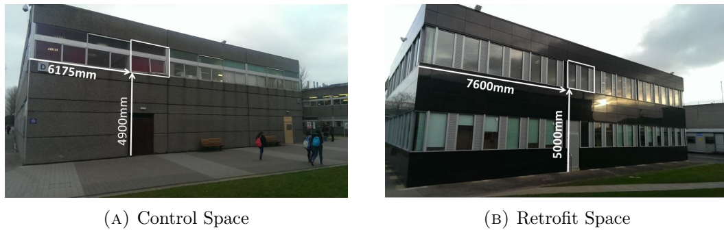
FIGURE 1.2: Control and retrofit spaces used for ACR and Internal Thermal Environment measuring campaign during summer 2013
