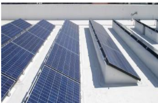
Fig 1.5: Fixing PV panels on flat roofs https://www.google.com/imghp
