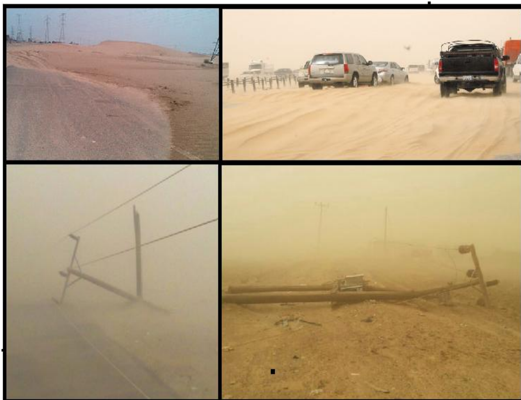
Fig 5.7: The Impact of sand dune encroachment and Sandstorms on the power transmission lines ( https://www.google.com/imghp )
