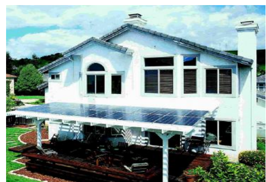
Fig 1.6: Using shade structures for mounting PV systems. https://www.google.com/imghp
