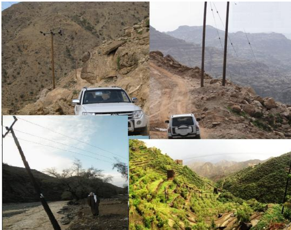
Fig 5.4: Electric poles in difficult topographies ( https://www.google.com/imghp )
