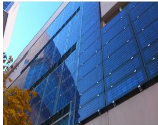
Fig 1.7: An example of BIPV system, where PV panels are used in the architectural and structural design. https://www.google.com/imghp
