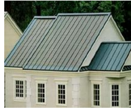
Fig 1.4: PV panels integrated with building https://www.google.com/imghp
