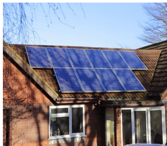
Fig 3.8: Shading occurring via trees, https://www.google.com/imghp
