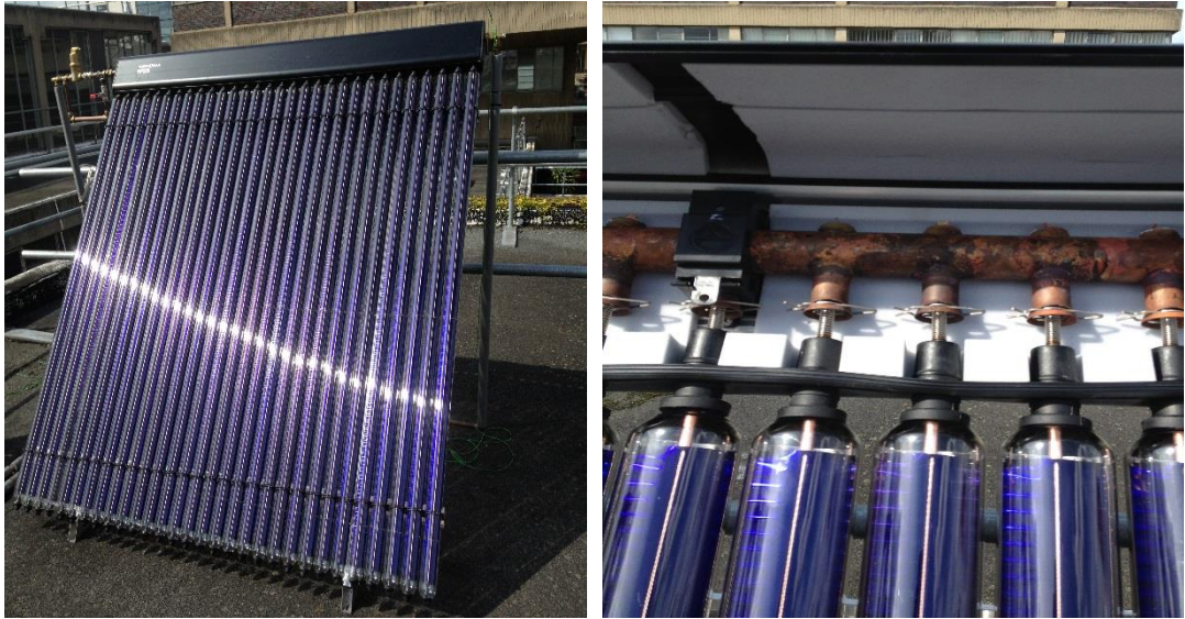
Figure 3.4. Evacuated Tube Collector
