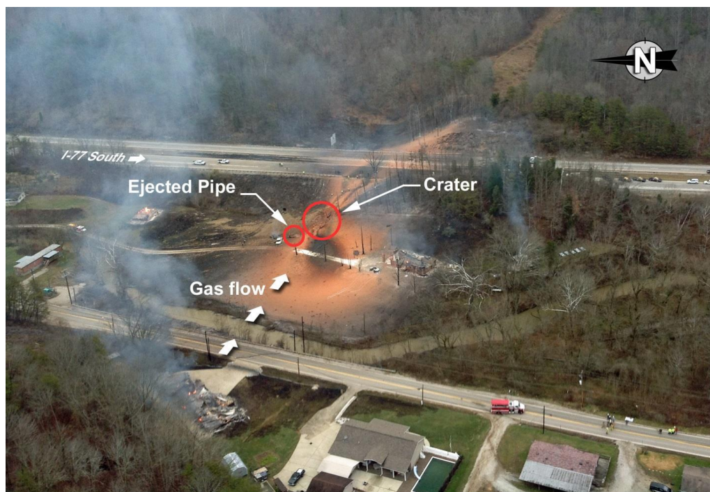
Figure 2-3. Columbia Gas Transmission Corporation pipeline rupture consequences [13]
