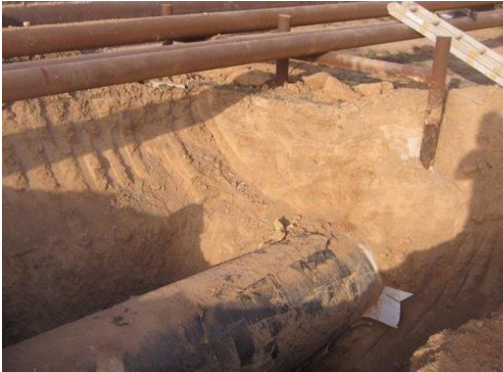
Figure 3-15. Example of pipeline close to pipe supports.
