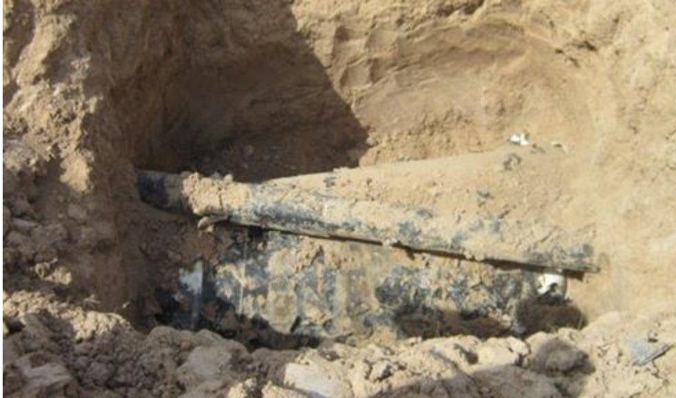
Figure 3-12. Example of pipelines crossing very close to each other.
