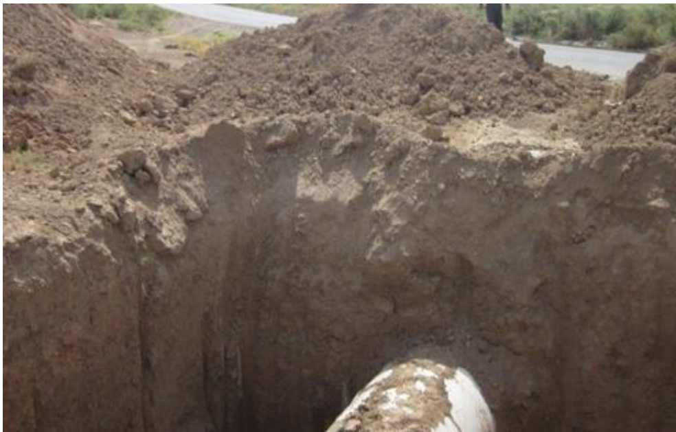
Figure 3-11. Example of a pipeline crossing a road.
