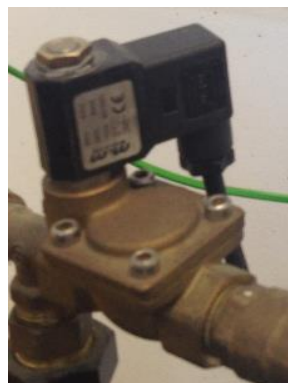
Figure 3-12. Solenoid valve used to control system cooling.
