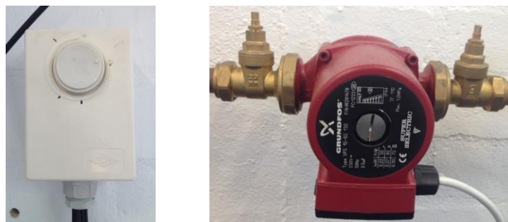
Figure 3-4. Voltage controller (left) and external pump (right).
