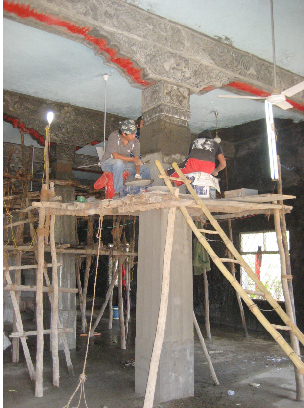
Fig. 6.5 Source: Author's own The workmen carving the temple columns
