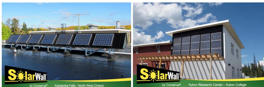
Figure 2-15: PVT Solar Duct left and PVT Solar Wall Right. Source Conserval Engineering
