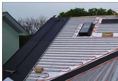
Figure 2-16: BIPVT water system. Source Englert [63]
