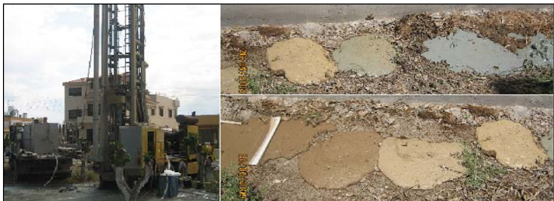
Figure 3.6: Drill chipping samples collected during drilling
