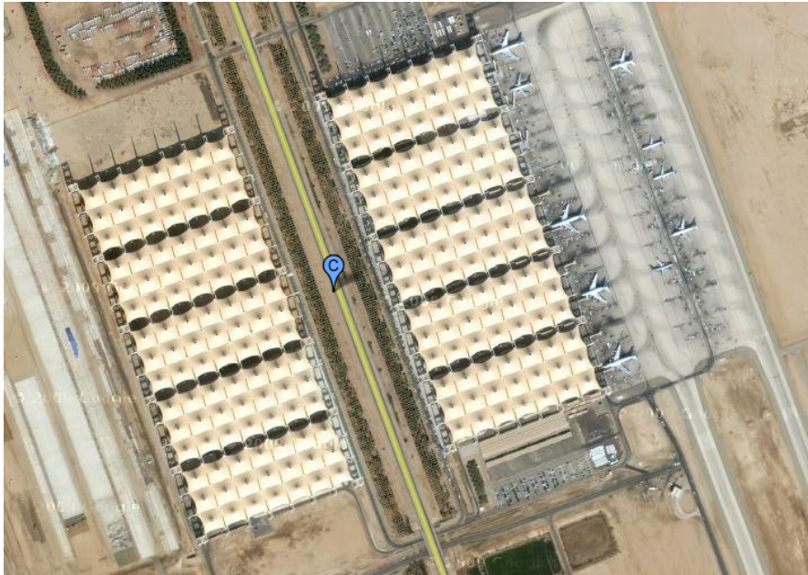
Figure 1.3 Google earth view of the Hajj terminal, showing the 5 running modules in the east portion of the Hajj terminal complex.
