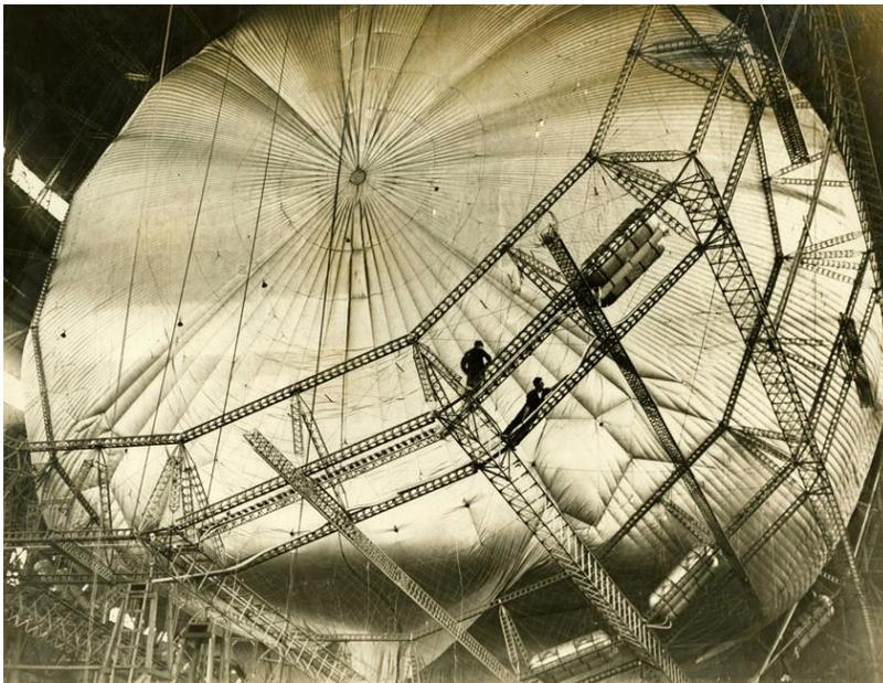
Figure 4, Inserting gas bags (believed to be) between R101B and R101C
