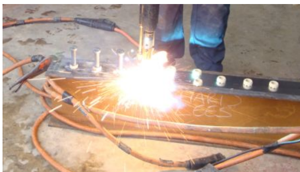
Figure 2 - Through deck welding
